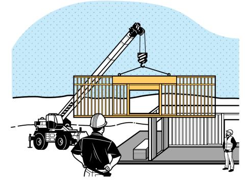
PREFAB WALL PANELS ARE SHIPPED TO THE SITE AND CRANED INTO PLACE.
